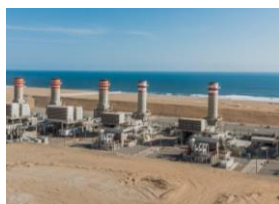
Ilo41 (2016, Nodo) • 610MW - Dual Fuel Ilo31 (2013, Reserva fría) • 500MW - Dual Fuel
